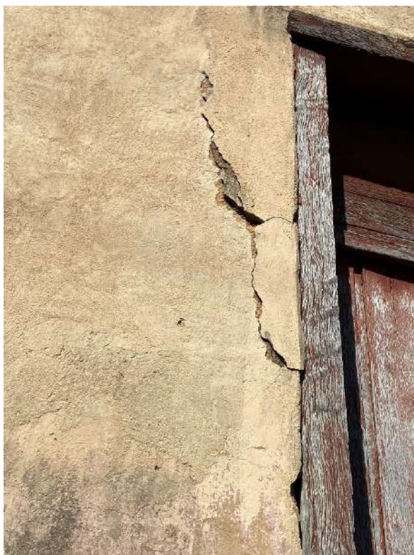
Figura 30.1 – Rachadura
